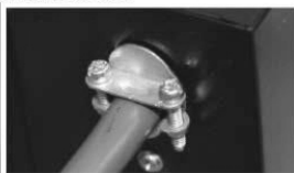
Figure 11: Installing cable fitting to heater
