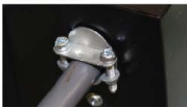
Figure 11: Installing cable fitting to heater
