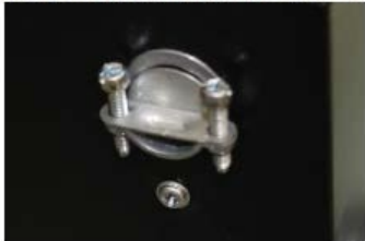
Figure 11: Installing cable fitting to heater
